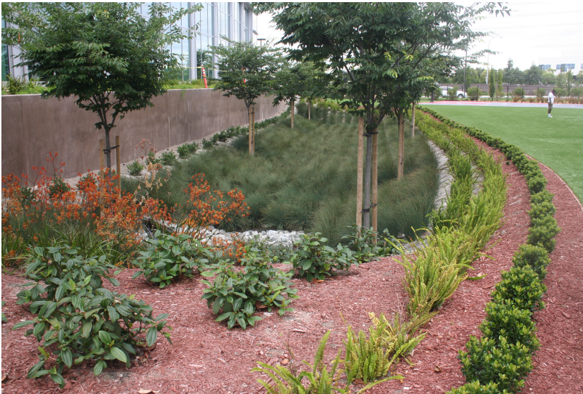
Figure 17: An image of a fully planted bioinfiltration swale -Wikimedia Commons – File:Bioswale @first.jpg.
