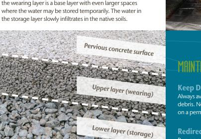
Newly installed permeable pavements can have tested infiltration rates of over 200 inches per hour! They can take a lot of stormwater. Over time, however, the pore space in these pavements may become impeded with sediment and debris which reduces the functionality of the pavements.
